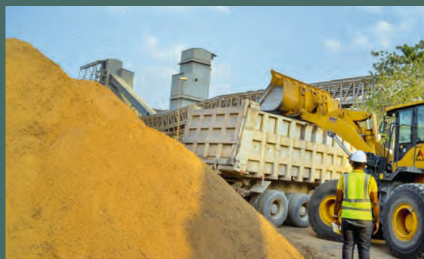
Stockpiling of agro-waste to be utilised as alternative fuel at the Obajana plant.
